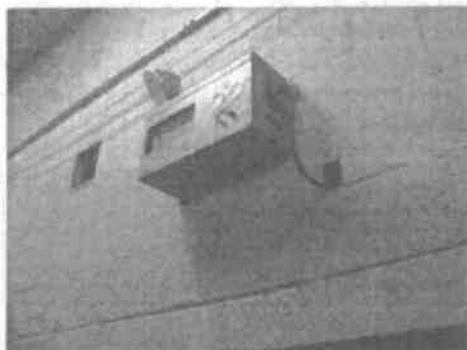
Figure 5 emergency lighting unit-ELU
