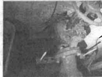
Figure 18 grounding electrode conductor
