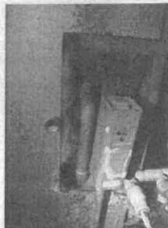
Observed rust at integral exchanger
