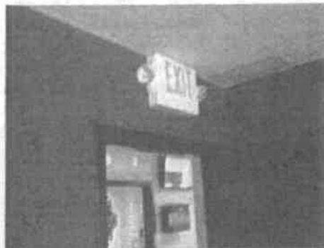
Figure 6 combination exit sign and ELU
